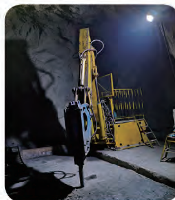
破碎机远程遥控系统 Crusher remote control system
