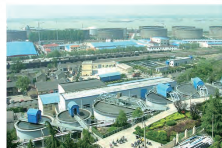
复杂金银多金属整体综合利用技术 Technology for comprehensive utilization of complex lead and zinc polymetallic ore
