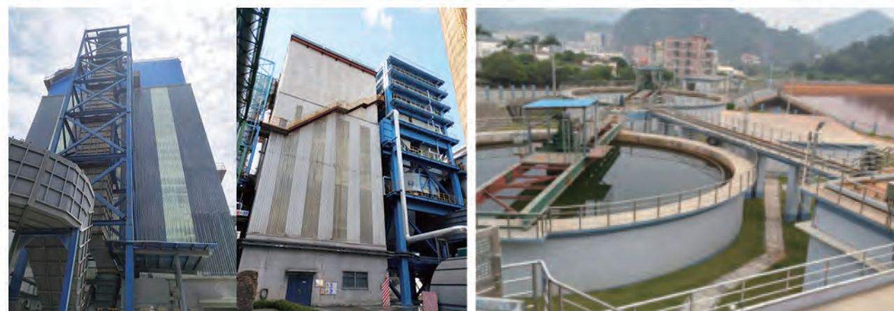
冶炼烟气脱硫脱硝工程 Smelting flue gas desulfurization and denitrification project
