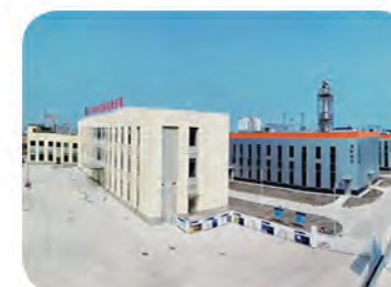
清洁高效选矿药剂研发与生产基地 R & D and production base of clean and efficient flotation reagents
