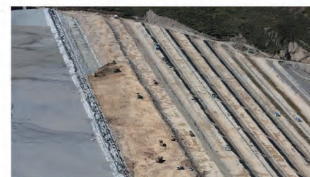
模袋法尾矿堆坝技术 - 西藏华泰龙矿业果郎沟尾矿库 Technology of tailings damming with geofabriform method--guolanggou tailings pond of huatulong mining in Tibet
